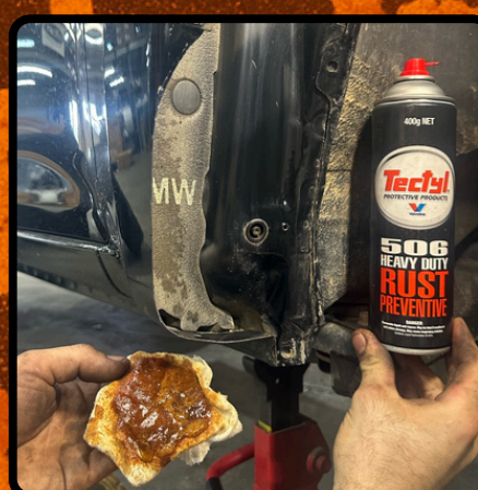
STEP EIGHT: Use a rust prevention spray on cut edges.
